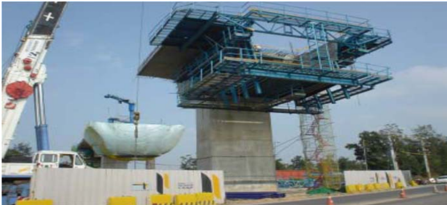
Figure 2. A suspension truss false-work system for the cantilever method
