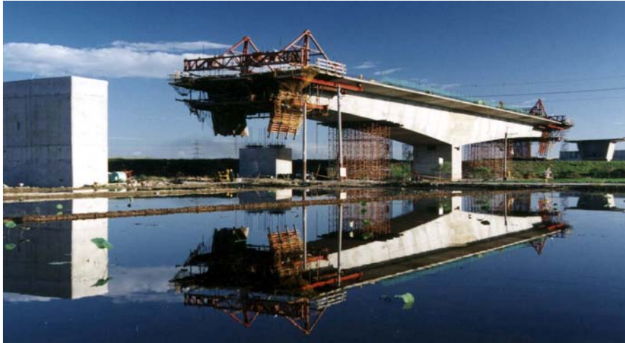
Figure 1. A cast-in-place cantilever bridge.
