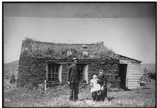
Figure 2. Sod roof in Milton, North Dakota, Norwegian Immigrant, c. 1896. Sod roofs were common in Norway because they added an additional layer of insulation and protection to the house.
