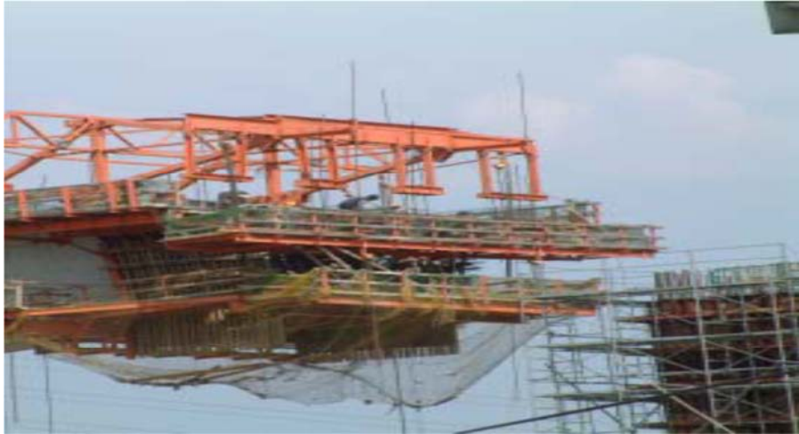
Figure 4. A diamond truss false-work system for the cantilever method
